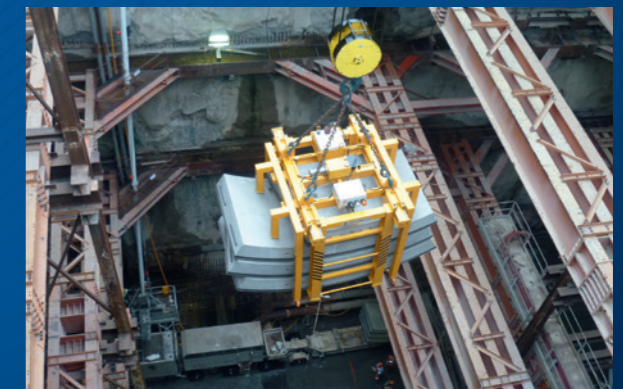
Self-powered hydraulic clamp
